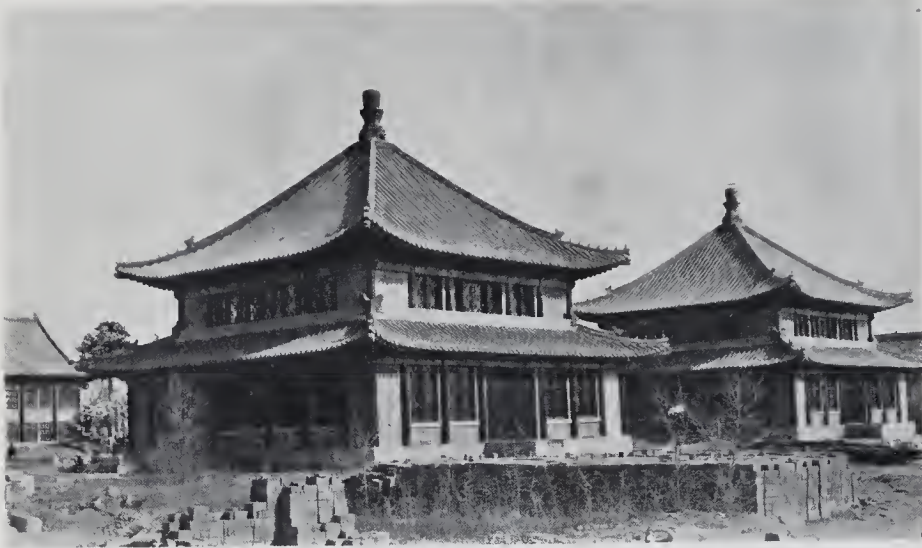
The "twins" of the Women's College—the Administration Building and Dean's Residence.
